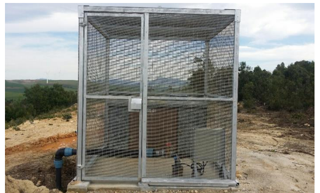
New Borehole – Caledon
